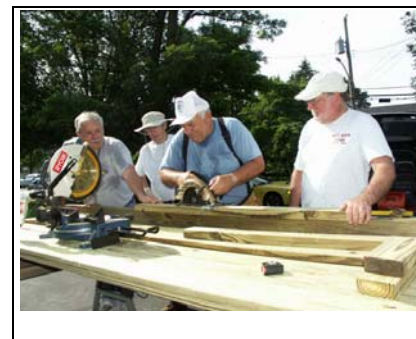
Massapequa Members Work on wheelchair ramp
